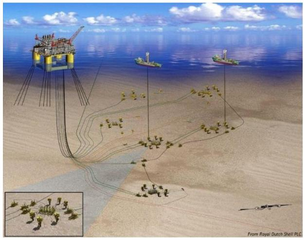
The Appomattox deepwater semisubmersible production platform will be located in 7,200 feet of water, 80 miles south of Mobile, Alabama. It will contain six drill centers, 15 producing sub-sea wells and five water injection wells.
